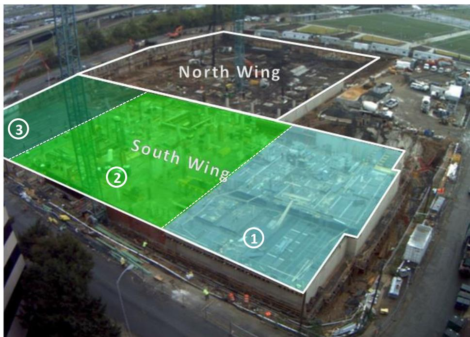
Figure 2 – Concrete Floor Sequencing Pours (Courtesy of Davis webcam)
